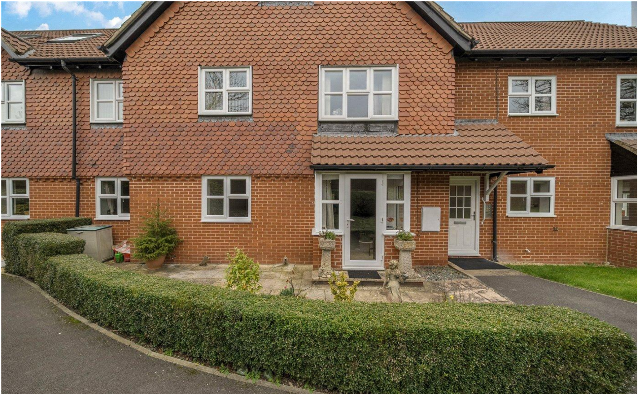
Apartment close to the High Street £249,000
