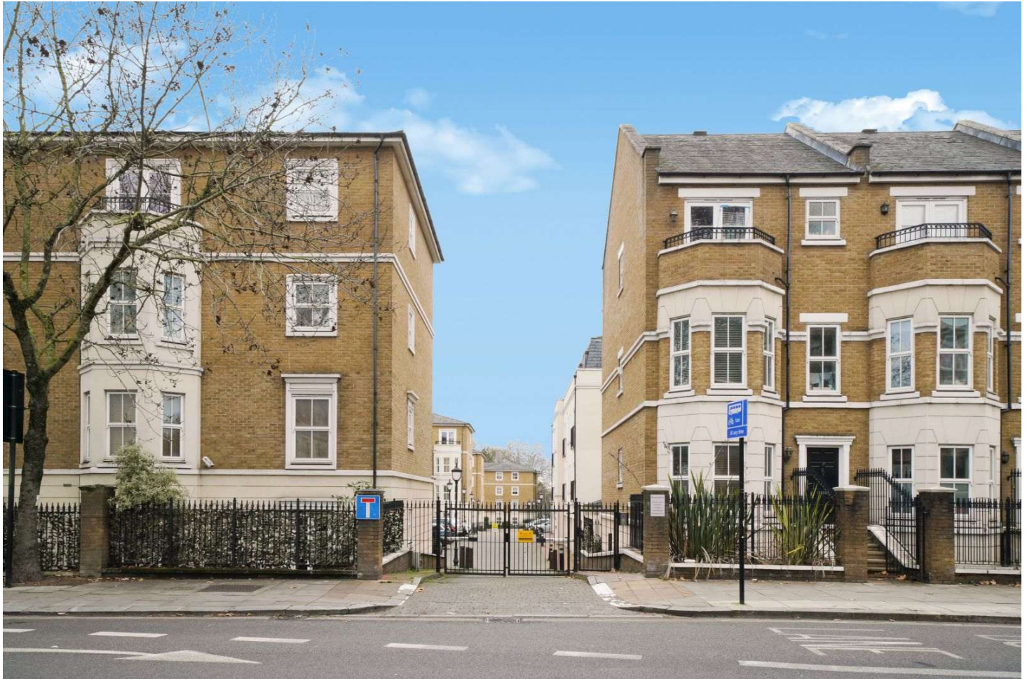
A view of a communal entrance
